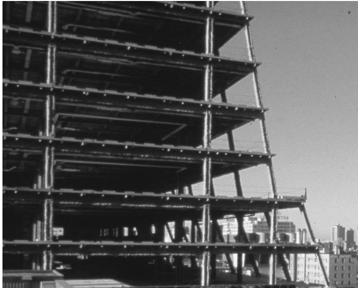
Figure 9 : vue d'une structure mixte, Thrivent Financial Building, Photo de City of Minneapolis Archives
